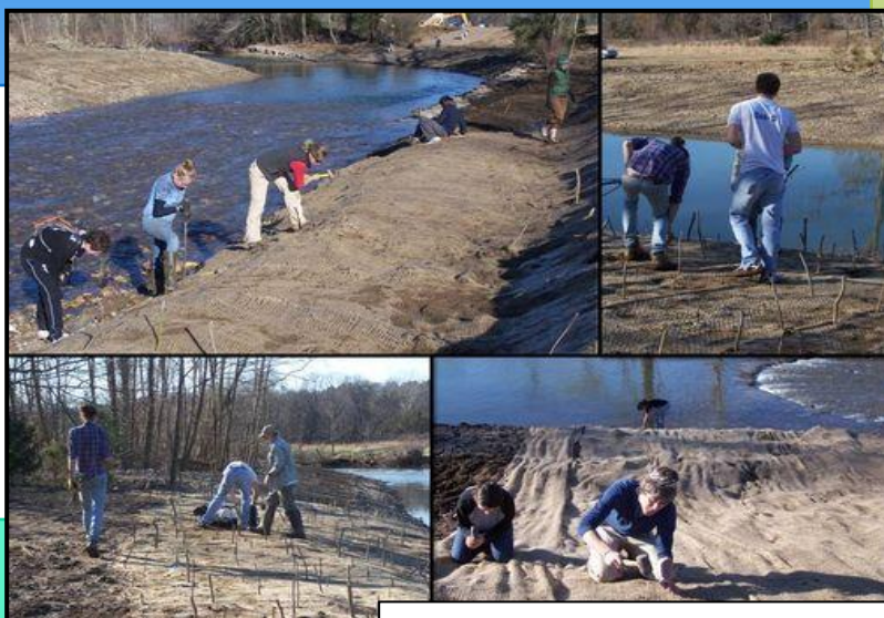
Repairing riparian area with erosion matting and tree cuttings
